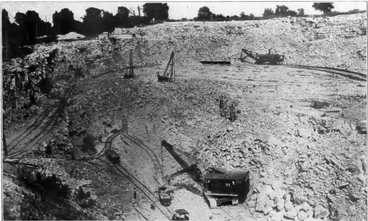
View of the Quarry Showing Track Layout
